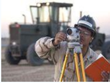
Dumpy level in use on a construction site
