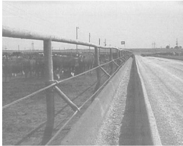
Feed Trough in a Double Row Arrangement
